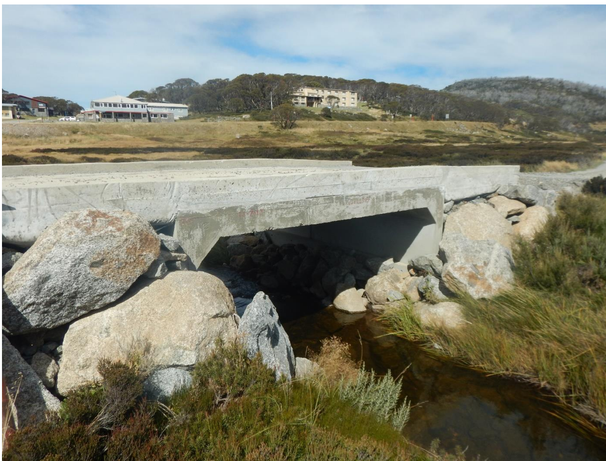
Photo 3: The existing open box culvert 750 m downstream.
