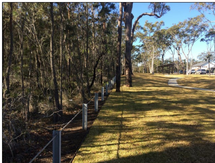
Figure 17: Example of bollards delineating cleared areas
