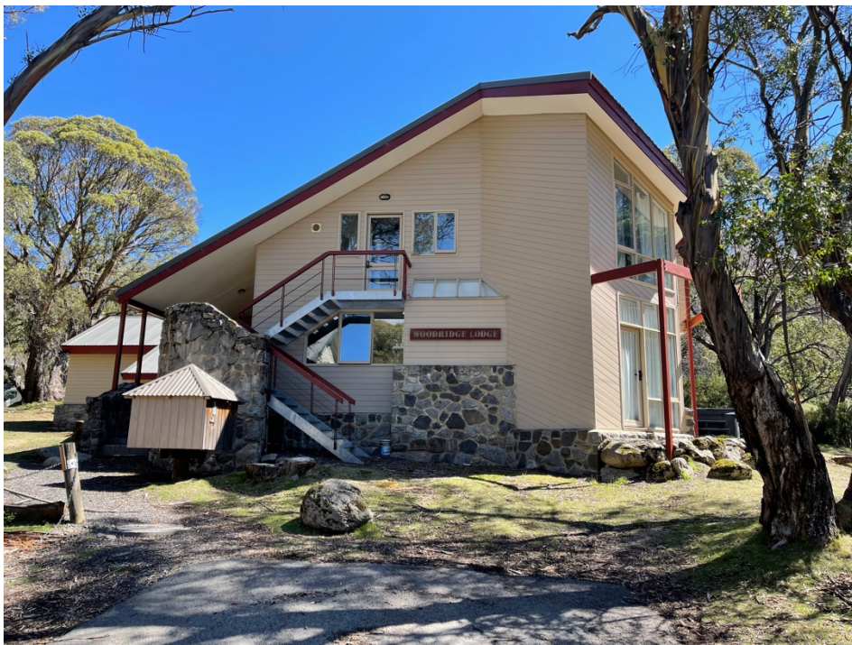
Photo 2 Continuation of Photo 1, looking west
