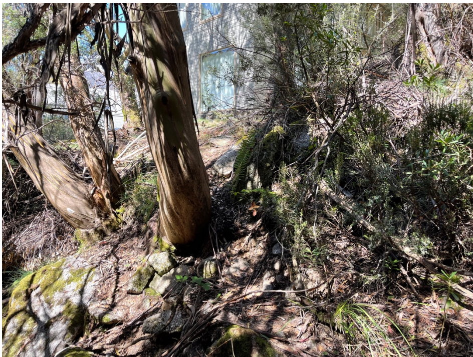
Photo 10 View of creek bank viewed from base of creek, existing lodge shown in background, looking approx. south
