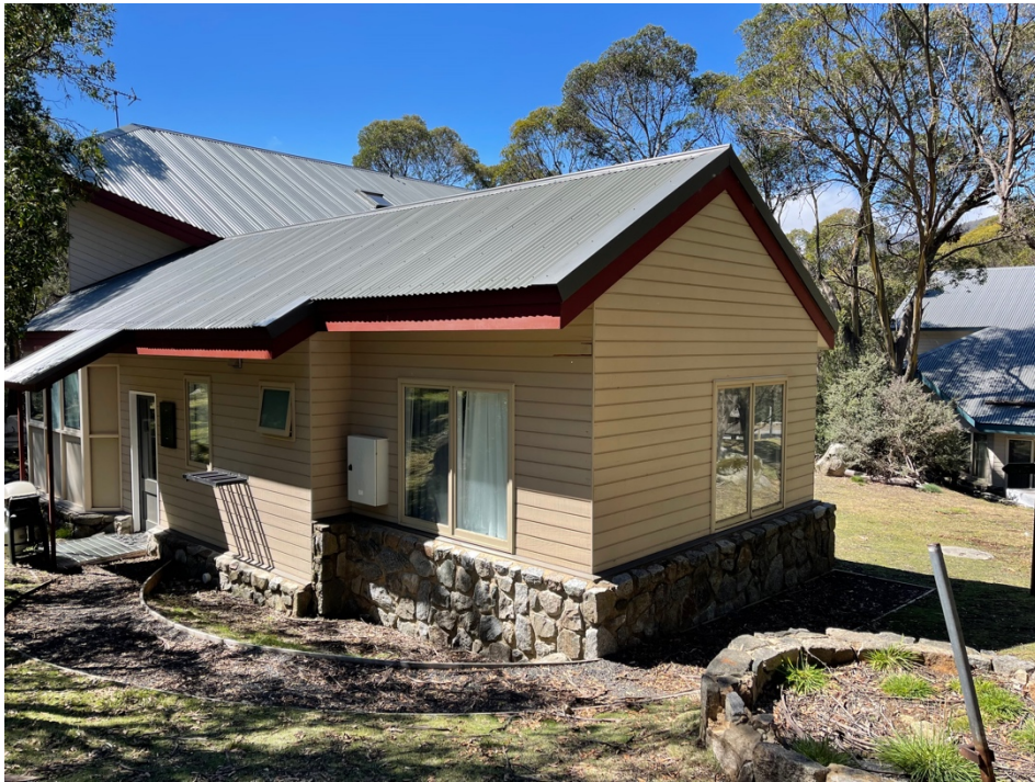
Photo 5 View of rear of lodge, looking north-east
