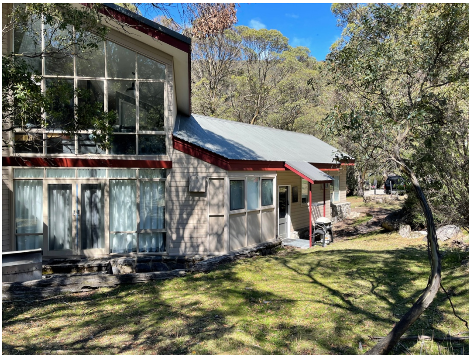
Photo 8 View of rear of lodge looking south-east (continuation of Photo 7)
