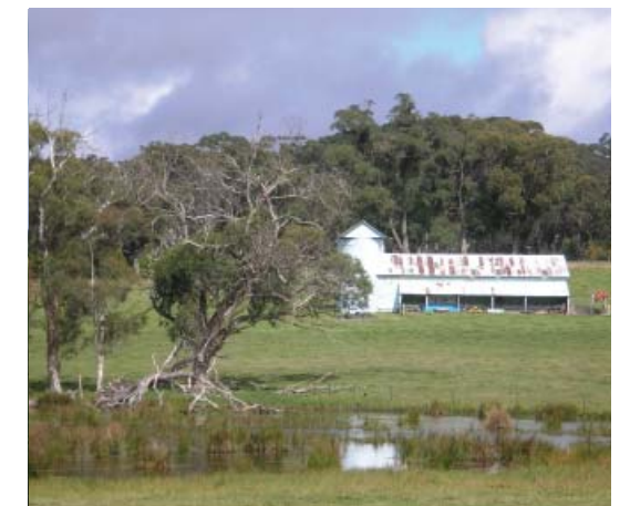
Typical rural shed
